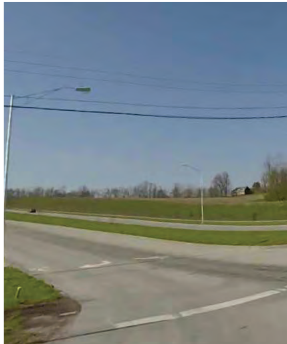
Polo Club Blvd at Winchester Road
