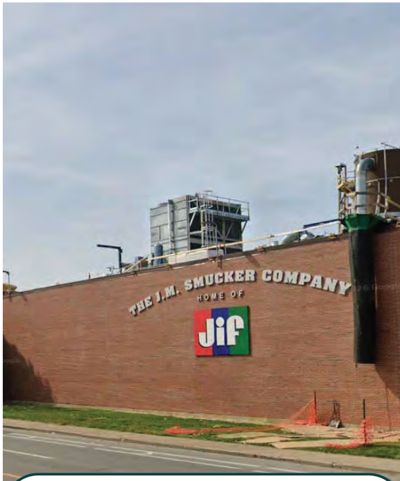
The J.M. Smucker Company Factory (JIF Plant)
