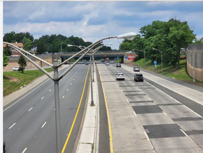
View of Route 440 from New Brunswick Ave (looking north)
