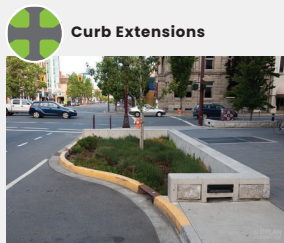
An extension of the sidewalk to narrow the street and shorten the length of the crosswalk.
