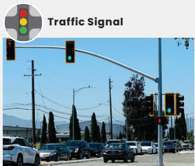
Assigns right-of-way at intersections and helps improves safety for all users.
