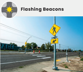
User-activated lights and signs that alert drivers when a cyclist or pedestrian is crossing.
