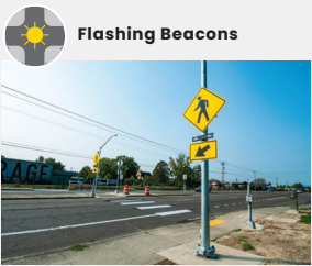
User-activated lights and signs that alert drivers when a cyclist or pedestrian is crossing is crossing.
